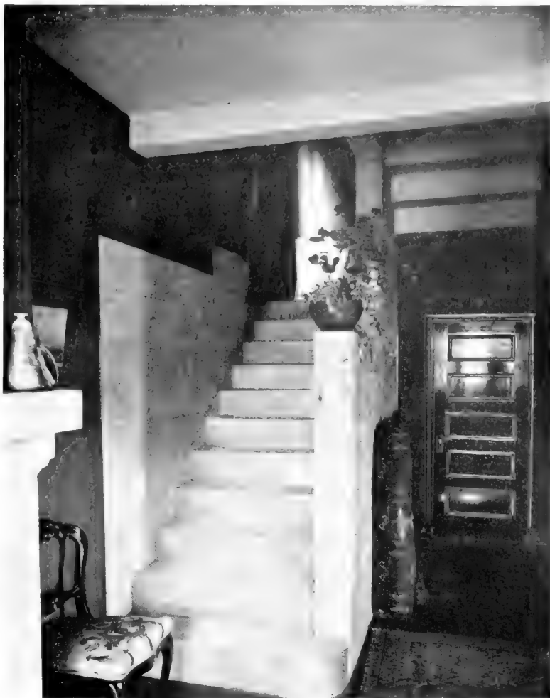
20—The Stairs and Hand-Rail are Built of Reinforced Concrete Treated with a Cement Tint
